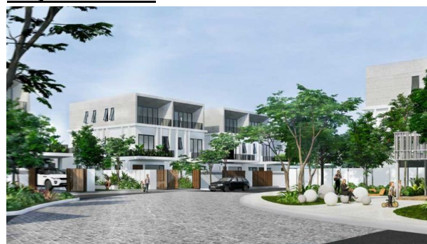
Chankiri Palm Creek gated-community project
