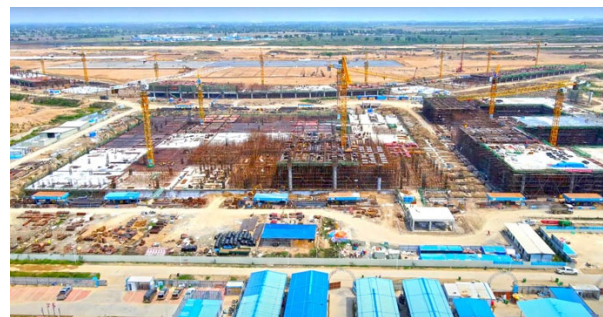
Construction Site of New Phnom Penh International Airport
