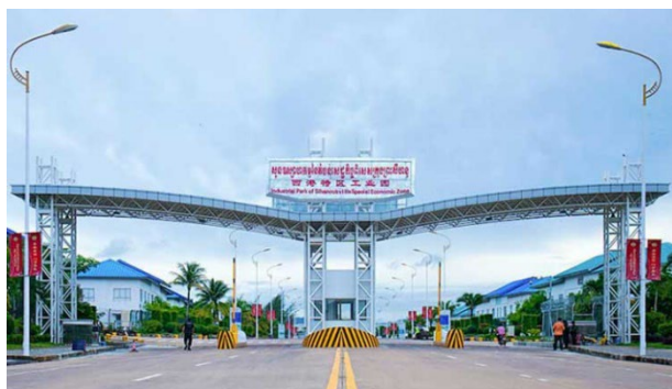
Industrial Park of Sihanoukville Special Economic Zone
