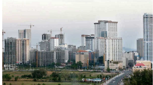
A view of under-construction buildings in Preah Sihanouk province in 2021.
