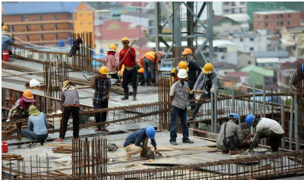
Building construction is underway at a site in Phnom Penh.
